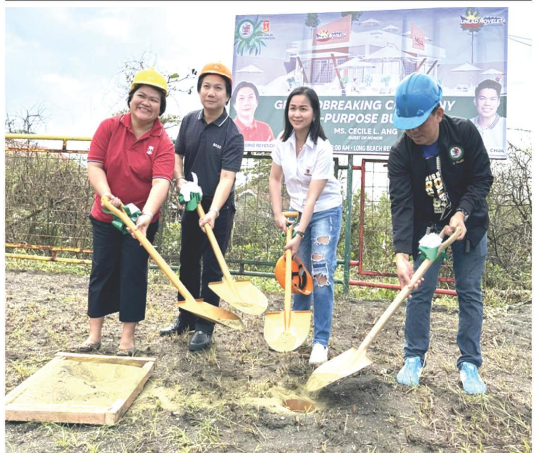
Ground-Breaking Ceremony of "unlaDCenter" Multi-Purpose Building na magsisilbi bilang Livelihood Training Center and Events Hall dito sa ating LONG BEACH RESORT & AQUA PARK with Ms. Cecile Ang, daughter of Mr. Ramon S. Ang (President and CEO of San Miguel Corp.)! This is a joint project of San Miguel Corporation and Local Government of Noveleta! #UnladNoveleta #UnladpaMore #SanMiguelCorp #LongBeachResort #LongBeachNoveleta #iloveNoveleta #unlaDCenter
